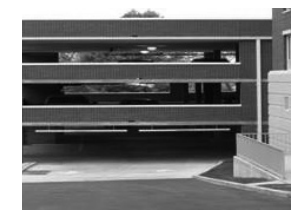
Four-level Parking Garage
